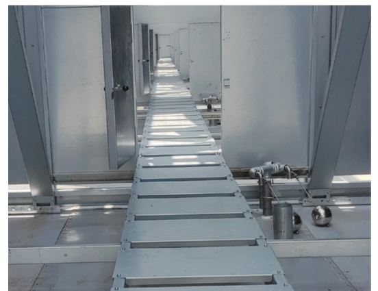
Inspection platforms in the tower
