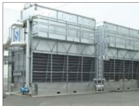
PCD Hood Installation
