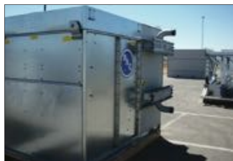
Cleanable Header Coil
