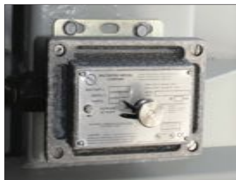
Vibration Cutoff Switch
