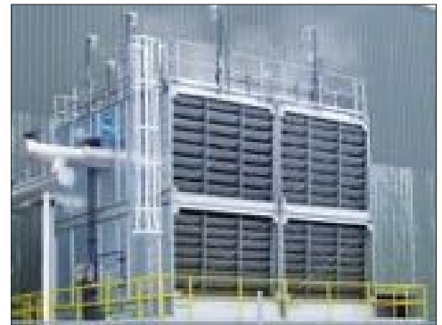
External Ladder, Safety Cage, and Handrail
