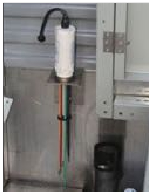
Electric Water Level Control
