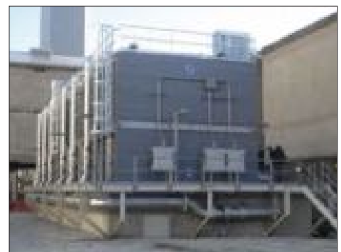
Flexible Piping Arrangement
